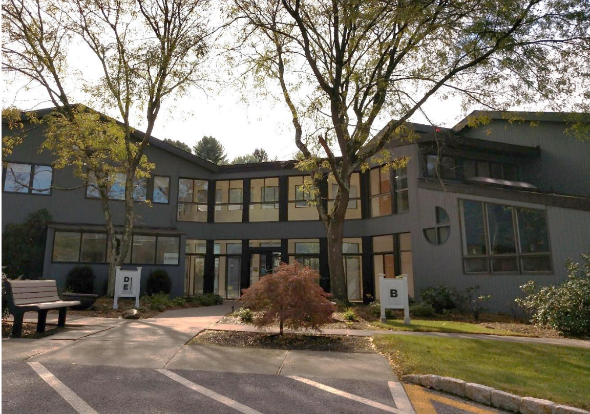
Photo 15: The medical complex buildings are all connected by enclosed walkways. View to the south.
