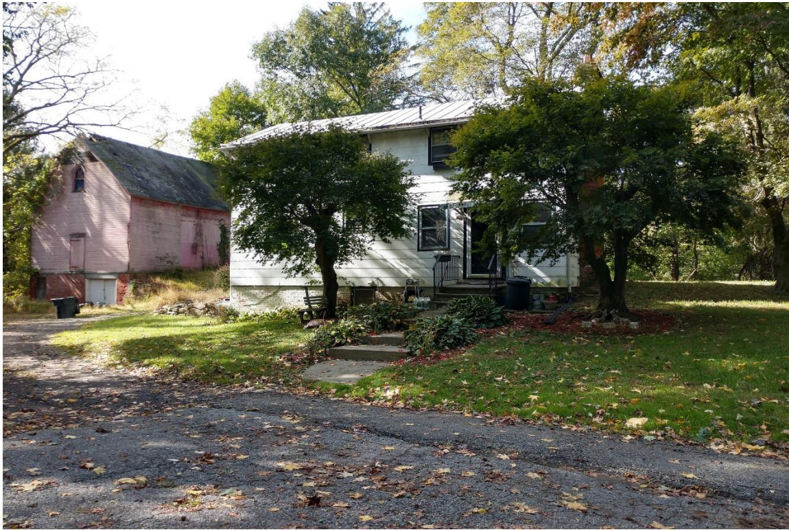
Photo 3: A residence and barn are located to the south of the Evergreen Manor structure. View to the southwest.
