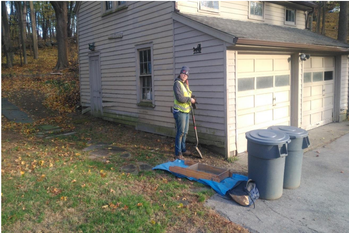
Photo 10: View to the south of the garage or carriage house located south of the Travis/Schumaker structure.
