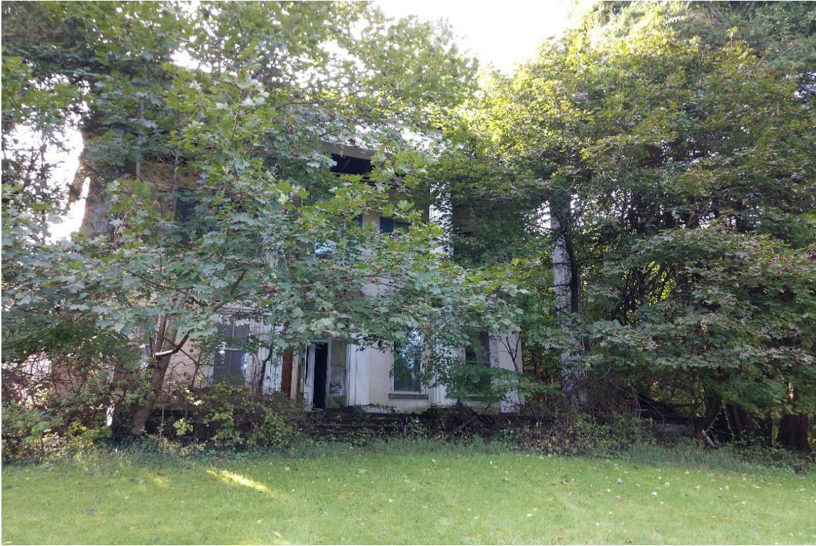
Photo 17: View to the south, of the former hotel building.
