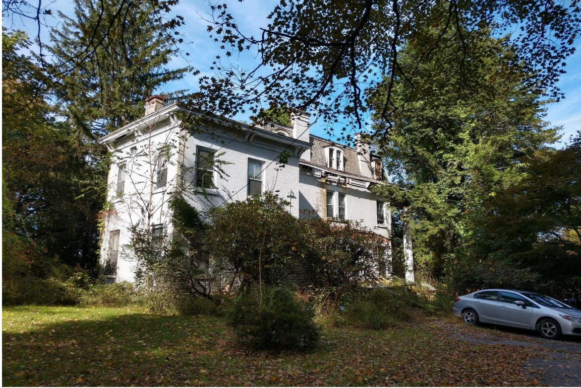
Photo 2: Evergreen Manor, a former hotel and Bed and Breakfast, is located in the center of the Project Area. View to the northwest.
