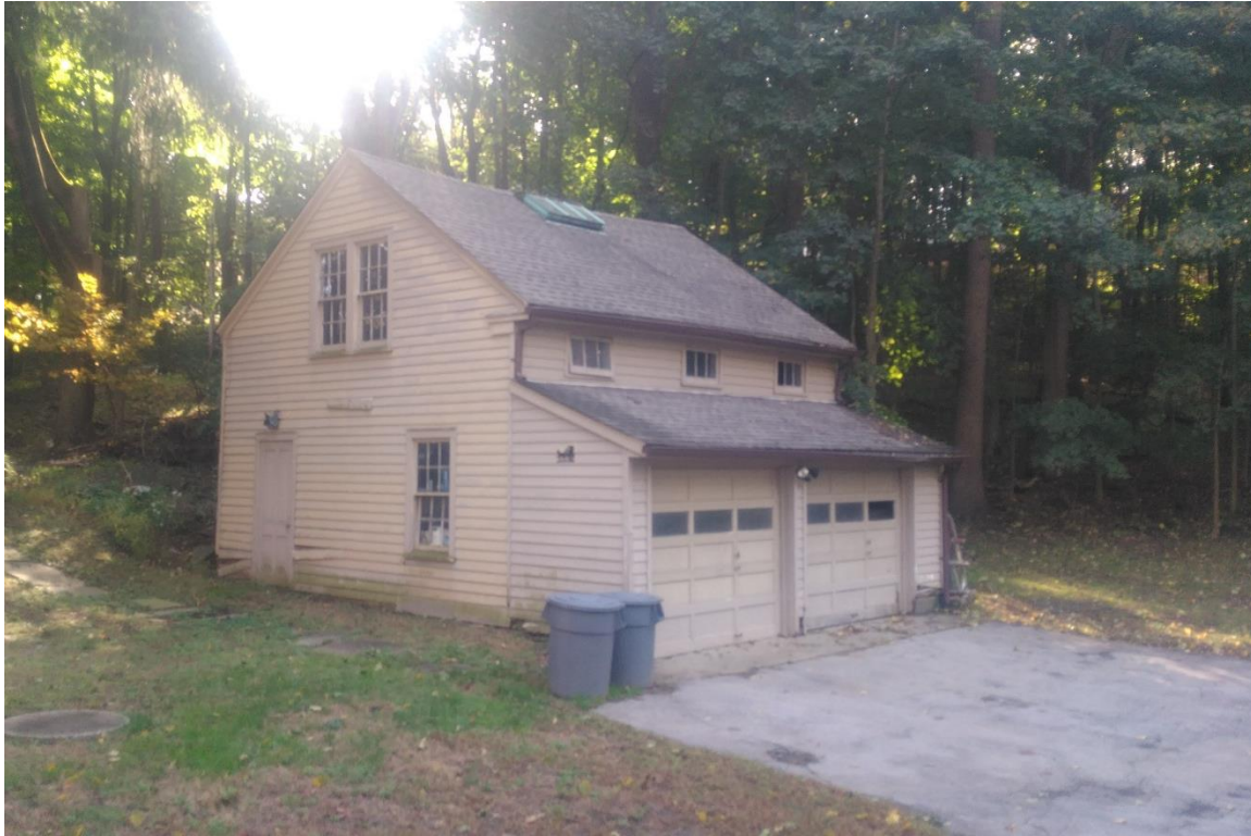
Photo 5: A two story wood frame garage is located to the south of the existing residential structures. View to the southeast.
